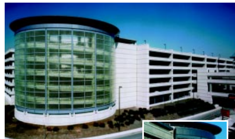
West Parking Garage Helix at Logan Airport | Boston, MA
