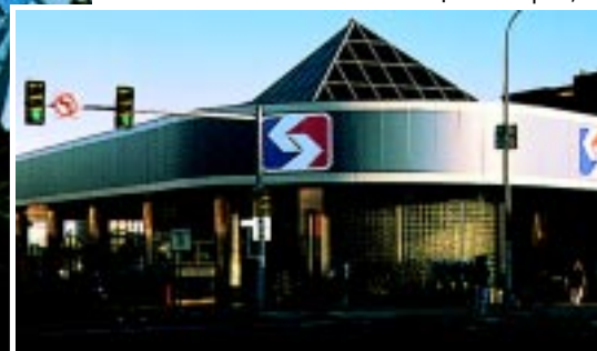
SEPTA Transit Station | Philadelphia, PA
