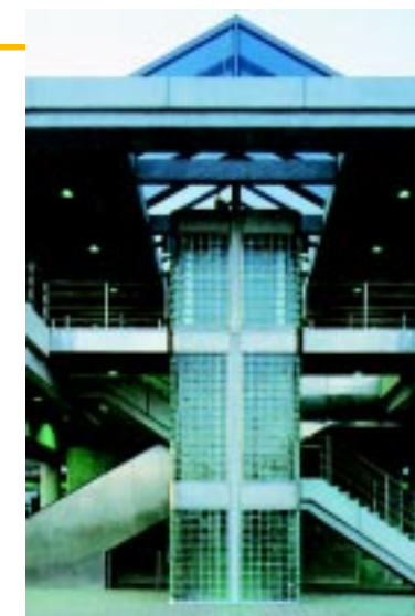
Miami Elevated Rapid Transit System | Miami, FL
